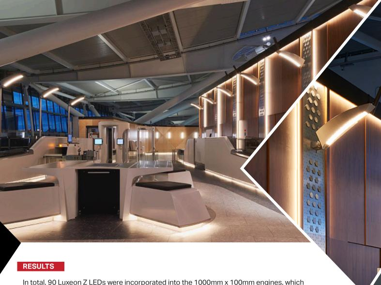
In total, 90 Luxeon Z LEDs were incorporated into the 1000mm x 100mm engines, which also had a micro-prismatic face to help diffuse the light. Each of the 14 wall and pole mounted luminaires were driven by a remote mounted 100W DALI dimmable driver.
