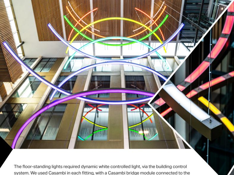
master system. Each fitting could then be placed anywhere with a power supply.
